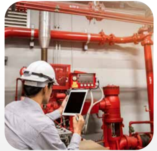
FIRE SUPPRESSION SYSTEM INSTALLATION
